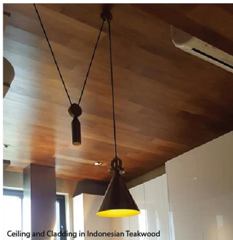
Ceiling and Cladding in Indonesian Teakwood
